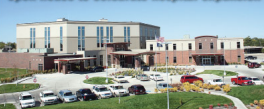
Community Health Center is set to open its new $10 million expansion project in Dodge City. The new building will provide more space for patient care, administrative offices, and support services.
