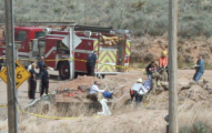
Workers are seen at the site of a body found under the Massoni Bridge on Road T in Liberal, Mo., on Friday, May 10, 2013. The body was found on the bridge deck. The bridge is a concrete structure with a steel truss design. The body was found in a shallow channel under the bridge. The area is surrounded by trees and a fence. The bridge is in the process of being replaced. The new bridge is a steel truss design. The old bridge is a concrete structure. The body was found on the bridge deck. The body was found on the bridge deck. The body was found on the bridge deck.
