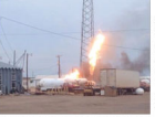
Elkhart authorities are investigating a propane blast that occurred at a propane storage facility in the city.
